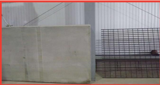
**9.** With the use of the M16 hex head and galvanised panel fixing cleat, secure the panel in place by threading the bolt into the cast in socket already cast into the back of the panel. Use a torque wrench to tighten up the fixing bolt.
