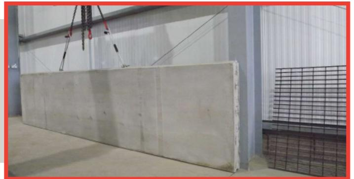
**8.** Ensure the panel unit is lined and level with the centreline of the steel column.
