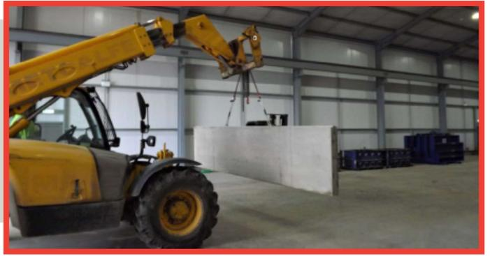
**6.** Approach the steel stanchions squarely and offer up the panel unit for installation, align the panel unit to the centreline of the steel upright. Check for alignment as you lower the panel unit slowly to the ground.
