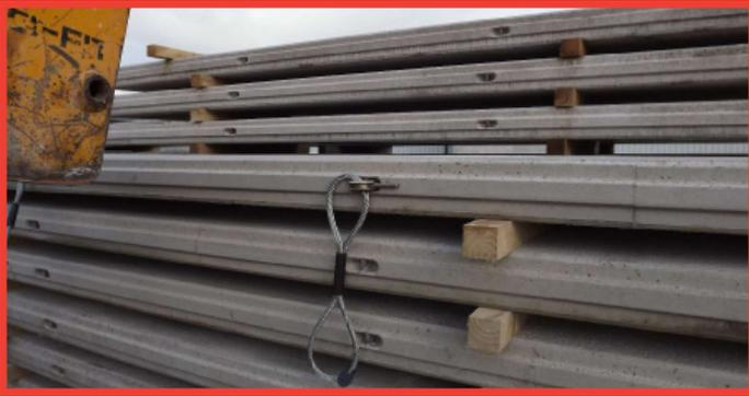
**2.** With use of 2.5t lifting clutch insert the cam into the embedded lifting eye and close the cam handle to the outside of the panel stack.
