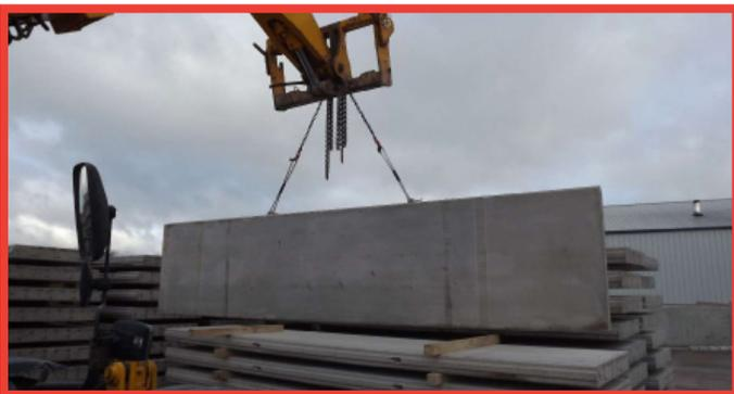
**4.** Slowly draw up the boom of the telehandler and lift the horizontal panel vertically upwards, take up the slack slowly as the panel becomes upright to avoid any swing.
