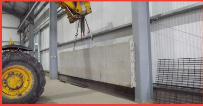
**7.** Lower the panel unit slowly to the ground checking for alignment as you go, keep the load secured by keeping a small amount of tension on the chains.
